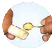
Solvent Cement Application
